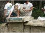
Set upper ledger piece 7; must be level from right to left but not critical from front to back. Set 8.
