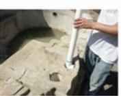
Drop PVC pipe in "pipe" column. Note threaded cap to allow pressure test.
