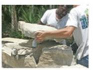
Mortar cap rocks 10 & 11 or use epoxy for less clean-up. Rake joints 1/2 inch after mortar sets.
