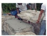
Set lower ledger piece 6 with mortar; match up column to column in base piece.
