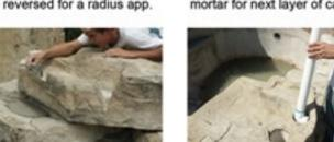
Set top basin piece 9 LEVEL, match pipe and lighting columns with lower level.
