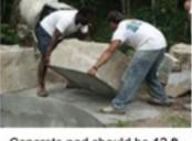
Concrete pad should be 12 ft. wide, 30" front to back. Dry set base pieces for alignment.
