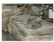
Use 1-2 inches of mortar for base pieces and 3/4 to 1 inch of mortar for next layer of castings.
