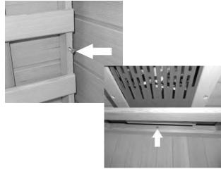
8. Attach the FRONT PANEL to the FLOOR. Buckle the FRONT PANEL to the LEFT and RIGHT PANELS.
