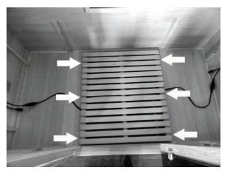
6. Slide each BENCH HEATER PANEL into place between the FRONT and BACK PANELS. Connect the heater plugs. Note: Make sure each FLOOR HEATER cable is placed through the groove in the bottom of the corresponding BENCH HEATER PANEL.
