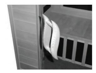
11. Attach the MAGAZINE RACK with 1-1/2" SCREWS. Attach the CUP HOLDERS with 3/4" SCREWS. Attach the DOUBLE TOWEL HOOK with 3/4" SCREWS.
