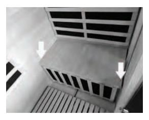
8. Lift the ROOF above the sauna, feeding the control panel and heater cables through the corresponding holes. Feed the cables for the MP3 PLAYER through the hole in the bottom of the ROOF. Secure the ROOF to the sauna with 1-1/8" SCREWS. Connect the control panel and heater plugs.
